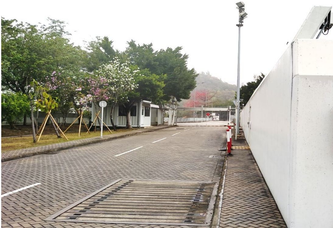
(17) This shows the thickness of the security wall provided
