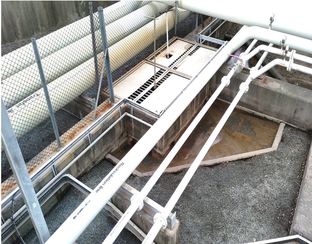
(19) Tank farm is with appropriate gradient and the drainage falls to interceptor for collection
