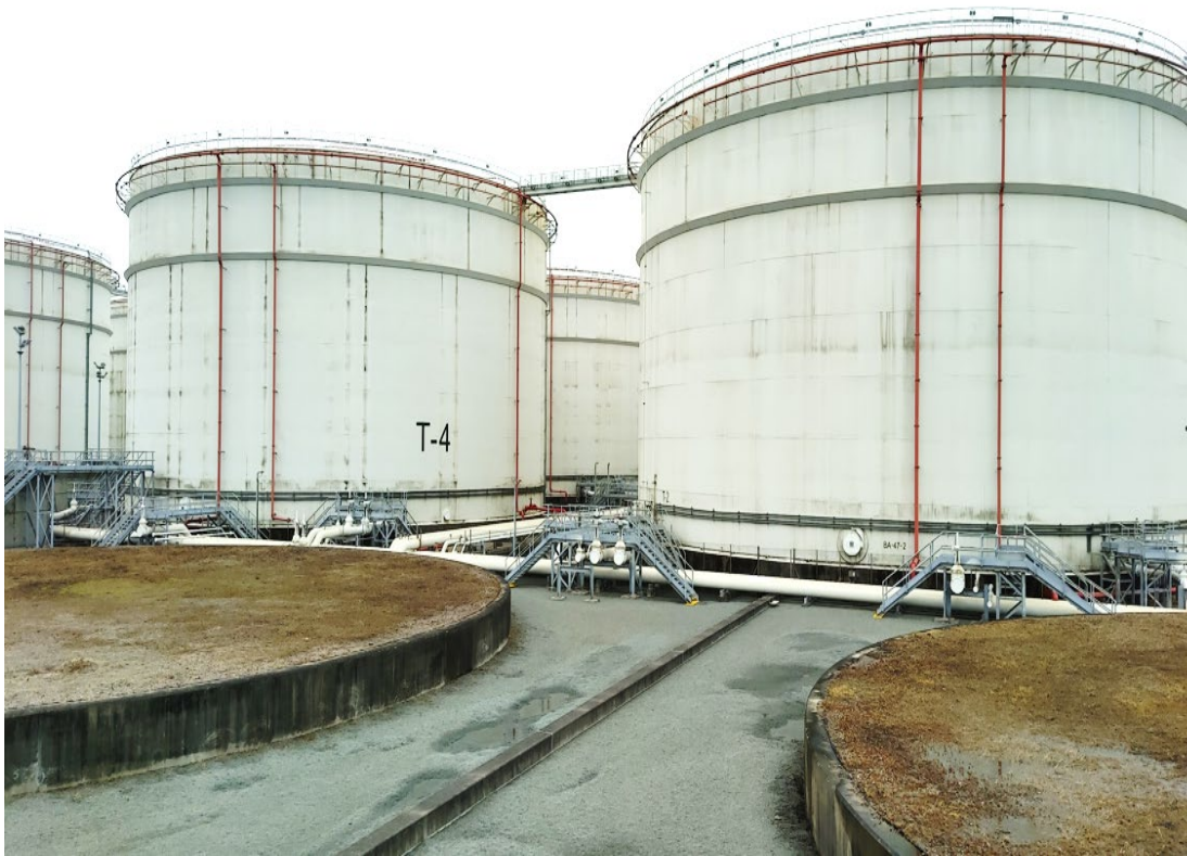
(1) Four tanks are located within bunded compound – Phase 1a
