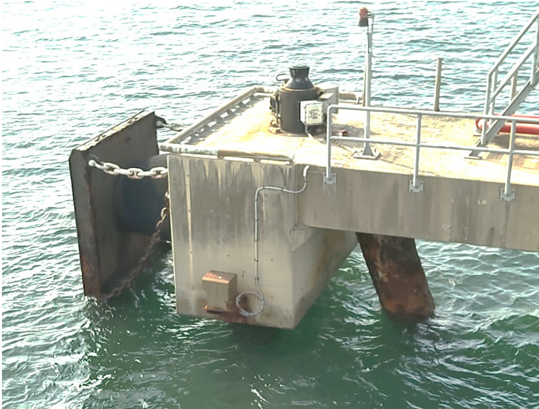
(37) Fenders are installed at sea side of the jetty
