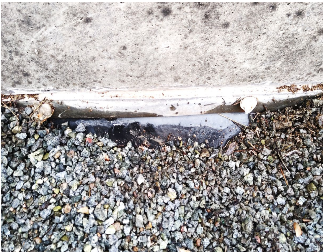
(18) Impervious lining are maintained in good condition
