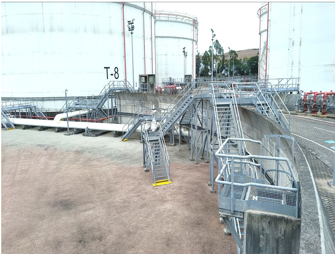
(4) Phase 1b bunded compound is lower than the ground level outside the bunds
