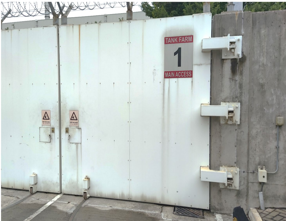
(14) Gates at security walls with sealant are maintained in good condition
