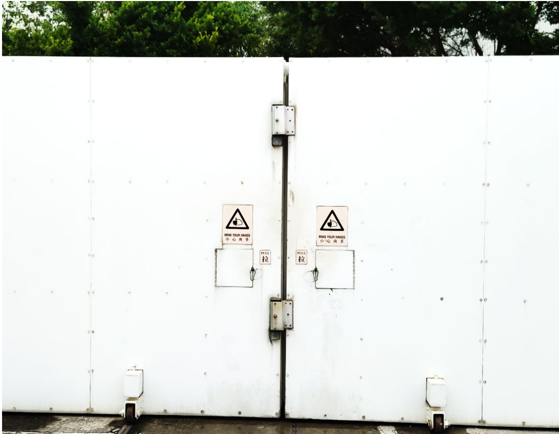
(15) Gates at security walls with sealant are maintained in good condition
