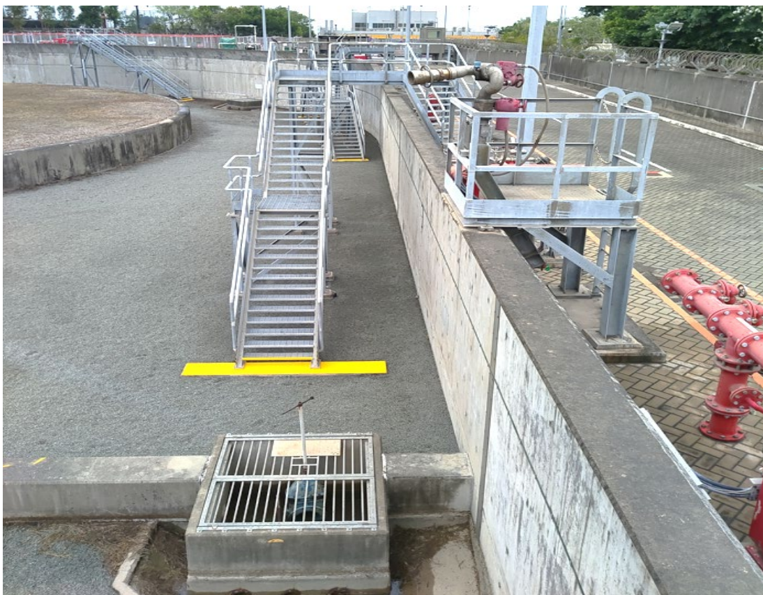
(16) This shows the thickness of the bund wall provided
