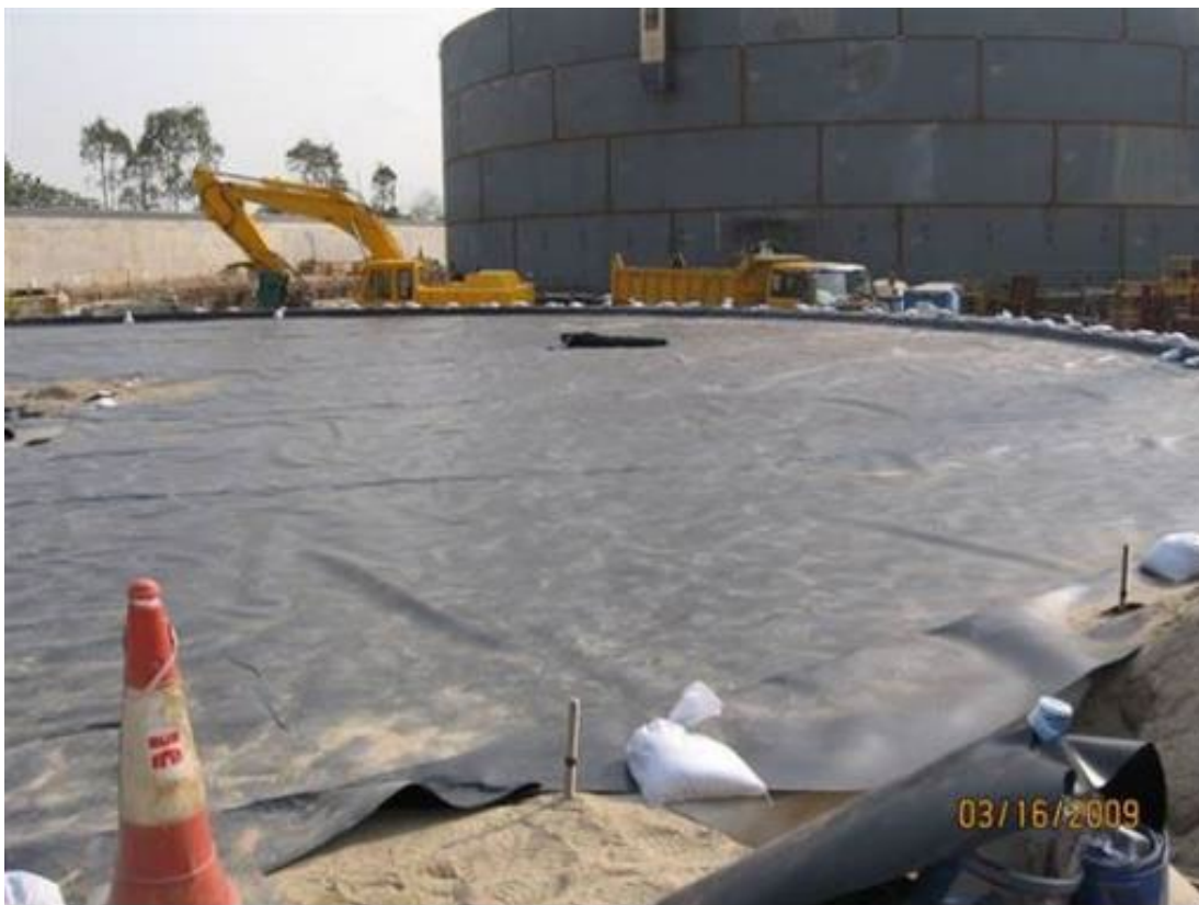
(22) Record photo shows impervious membrane being installed on top of tank foundation
