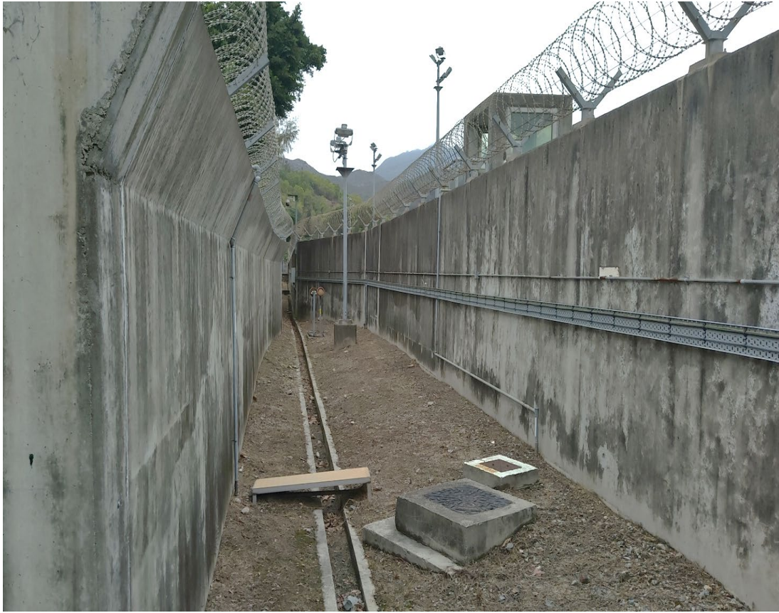
(11) Two impervious security walls are provided outside the bunded compounds
