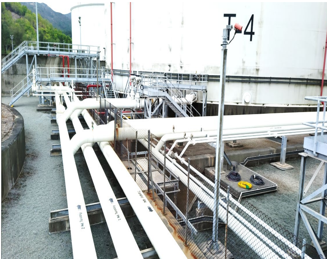
(8) Intermediate bund walls are provided in place near T-01-004
