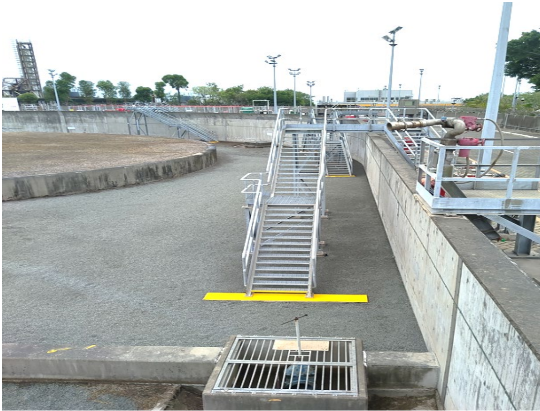
(3) Phase 1a bunded compound is lower than the ground level outside the bunds
